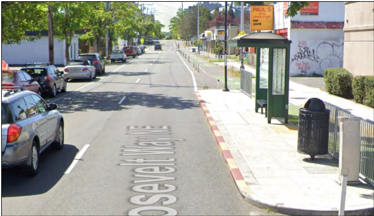
Figure 1-5. Existing Transit island/PBL configuration on Roosevelt Way NE
